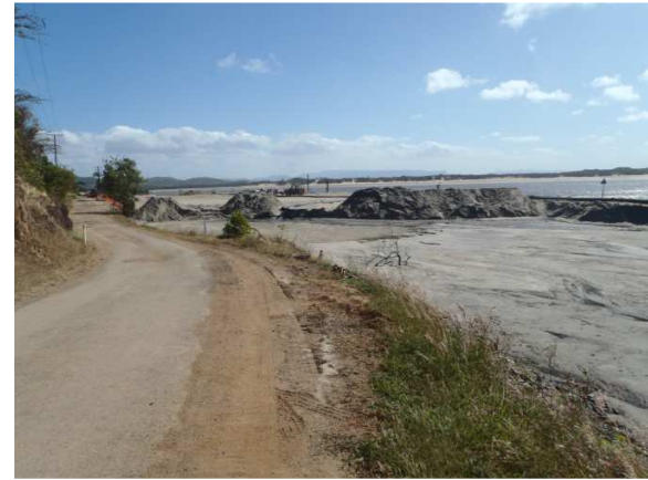
Sand pumping progress at 11/08/14
