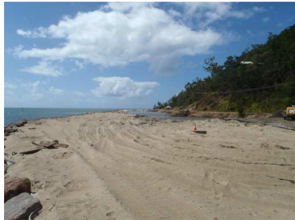
Sand backfill around tidal pool area
