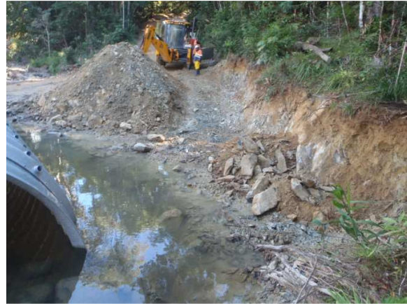
Excavation for wingwalls - Cairns side
