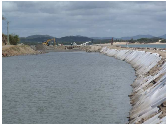
Geo Textile Fabric in place
