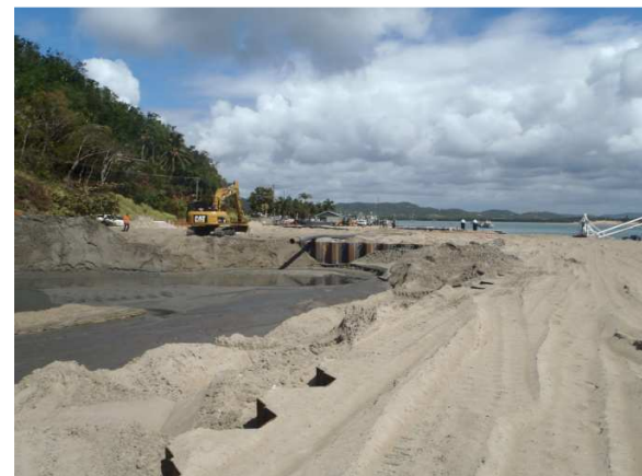
Pumping sand east of tidal pool area
