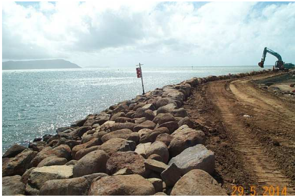
Landward end of rock wall completed
