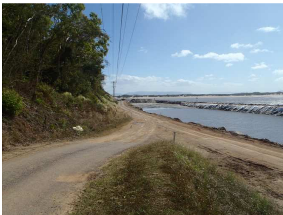
Sand pumping progress at 11/08/14
