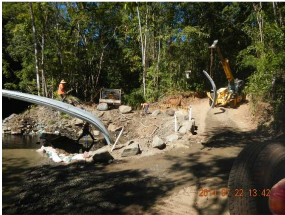
Culvert being put together
