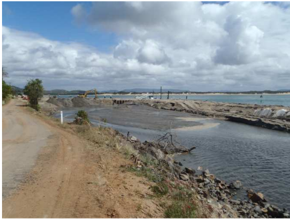
Sand pumping progress at 30/07/14
