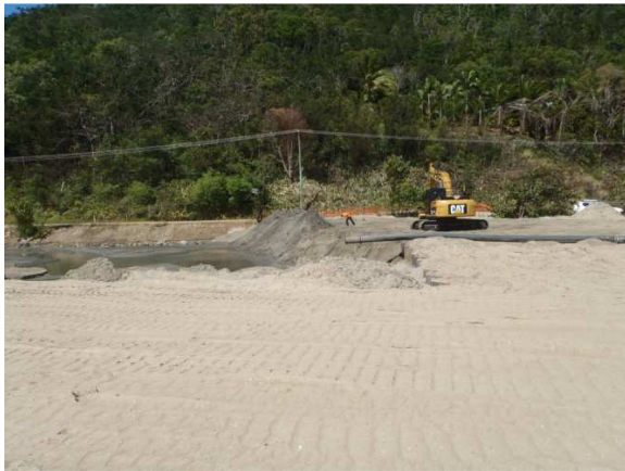
Sand backfill around tidal pool area
