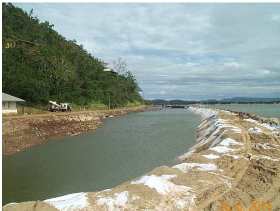
Geo Textile Fabric in place
