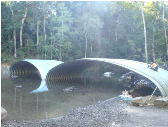
4000 bolts being tightened
