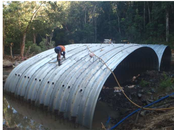
4000 bolts being tightened
