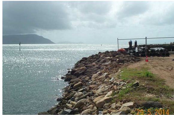
Tie in of 2 rock walls landward end
