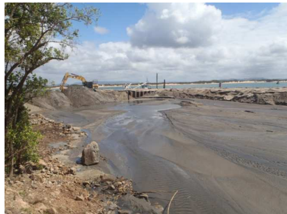
Pumping sand east of tidal pool area
