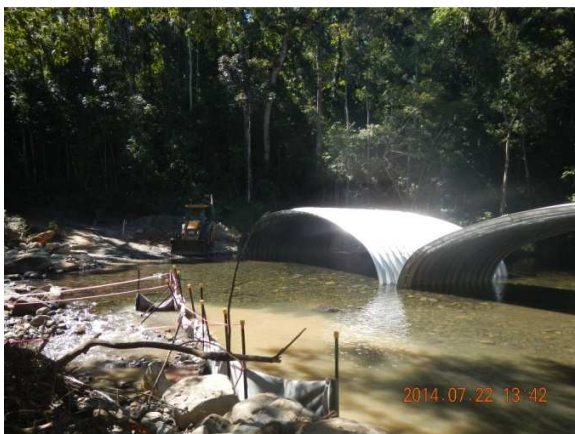
Silt trap protection of frog habitat
