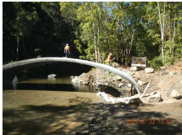
Culvert being put together
