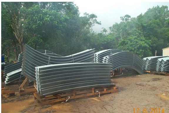
Culvert plate sections at CSC depot
