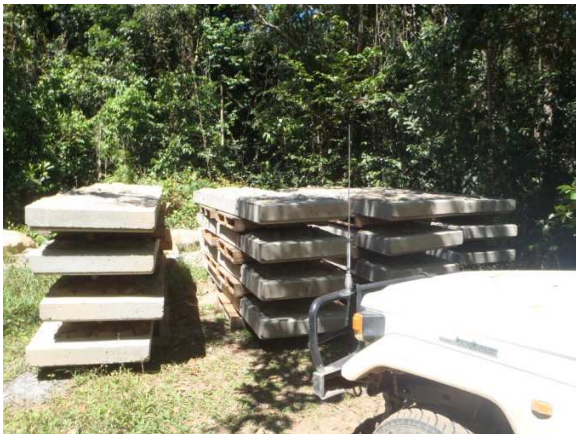
Link slabs & I-Beams for Wingwalls stockpiled on site
