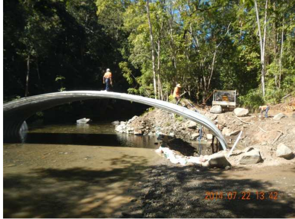
Culvert being put together
