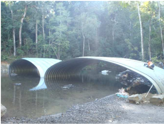
4000 bolts being tightened
