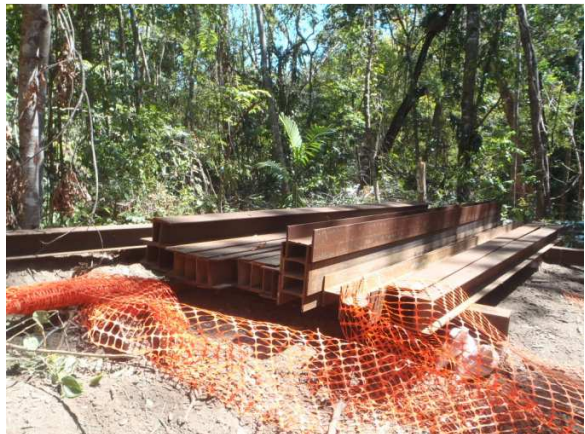
Link slabs & I-Beams for Wingwalls stockpiled on site
