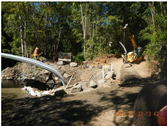
Culvert being put together
