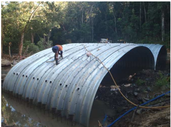
4000 bolts being tightened
