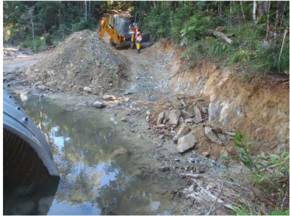
Excavation for wingwalls - Cairns side
