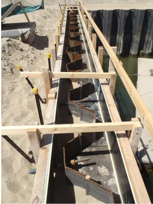
Concrete Collar formwork
