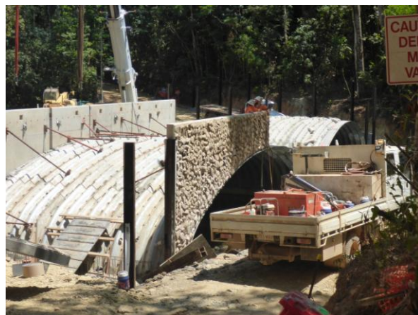
Placing headwalls upstream side
