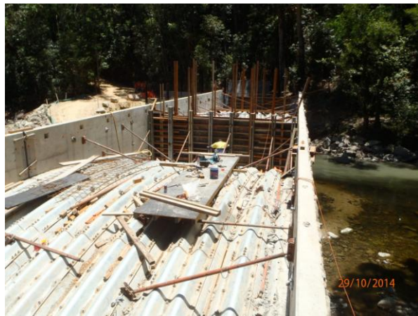
Centre sheerwall formwork
