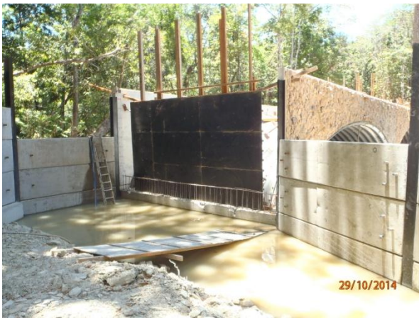
Cairns side sheerwall formwork
