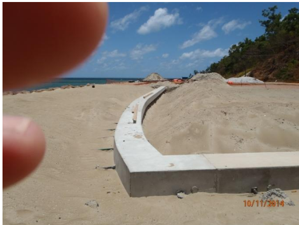
Tidal pool concrete capping completed
