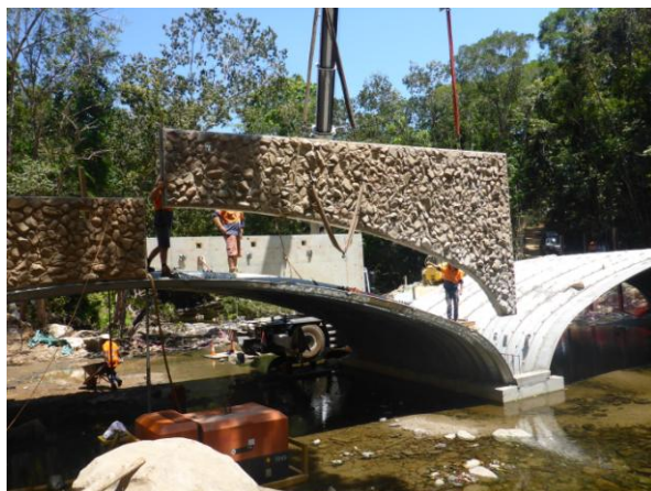
Placing headwalls upstream side
