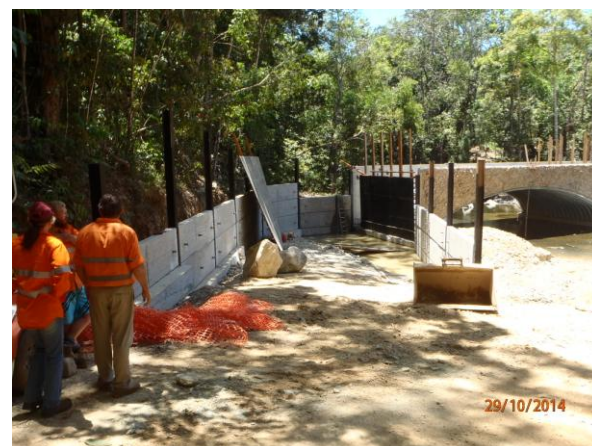
Down stream headwalls placed
