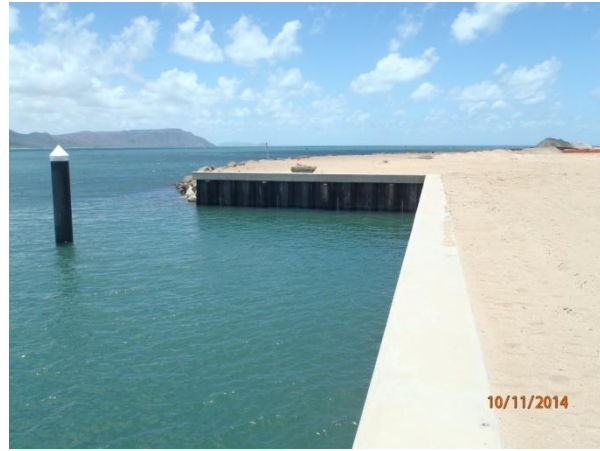
Boat Pen concrete capping completed
