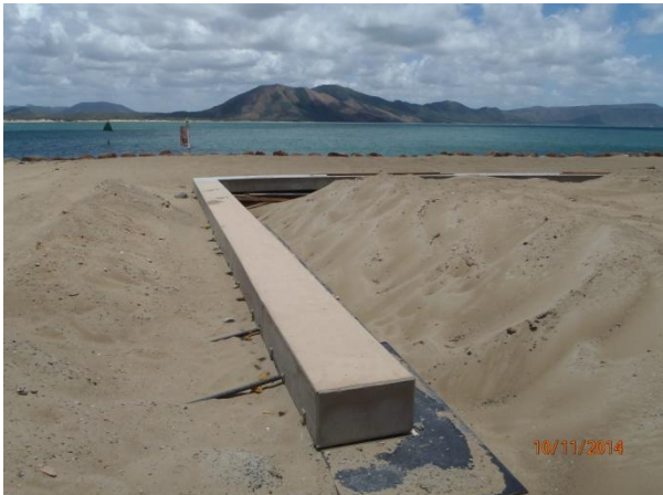
Tidal pool concrete capping completed
