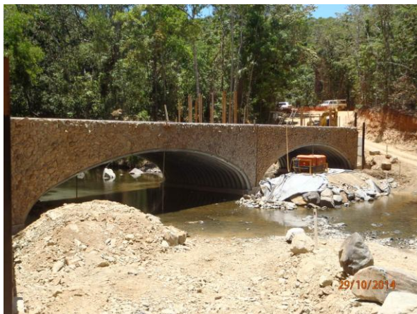
Down stream headwalls placed
