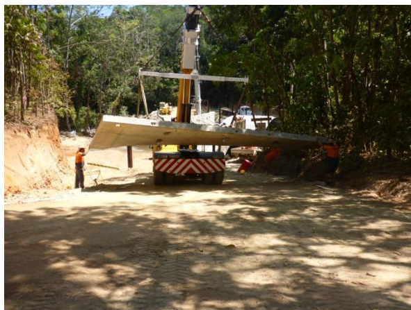
Transporting a headwall section
