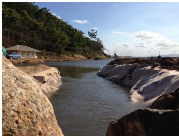
Drain through rock wall to lower water levels when backfilling
