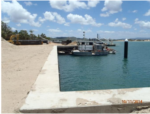
Boat Pen concrete capping completed
