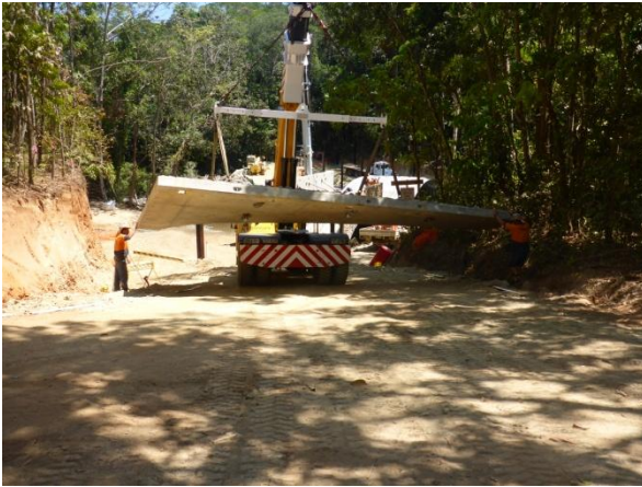
Transporting a headwall section
