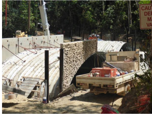
Placing headwalls upstream side
