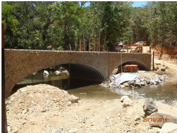
Down stream headwalls placed
