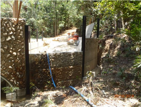
Cairns side wingwalls
