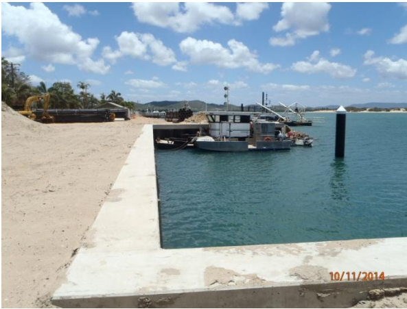
Boat Pen concrete capping completed
