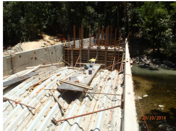
Centre sheerwall formwork
