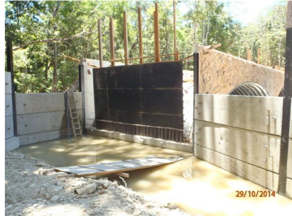
Cairns side sheerwall formwork
