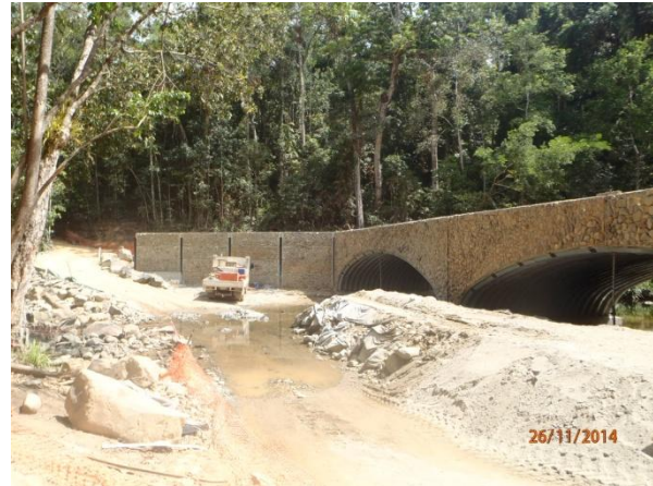
Cairns side approach-2 more sets of panels req'd to complete Cairns side windwalls
