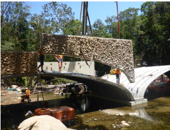
Placing headwalls upstream side
