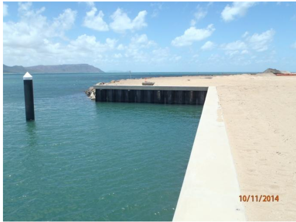
Boat Pen concrete capping completed
