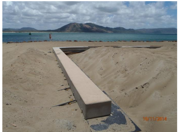
Tidal pool concrete capping completed
