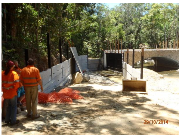
Cairns side wingwalls
