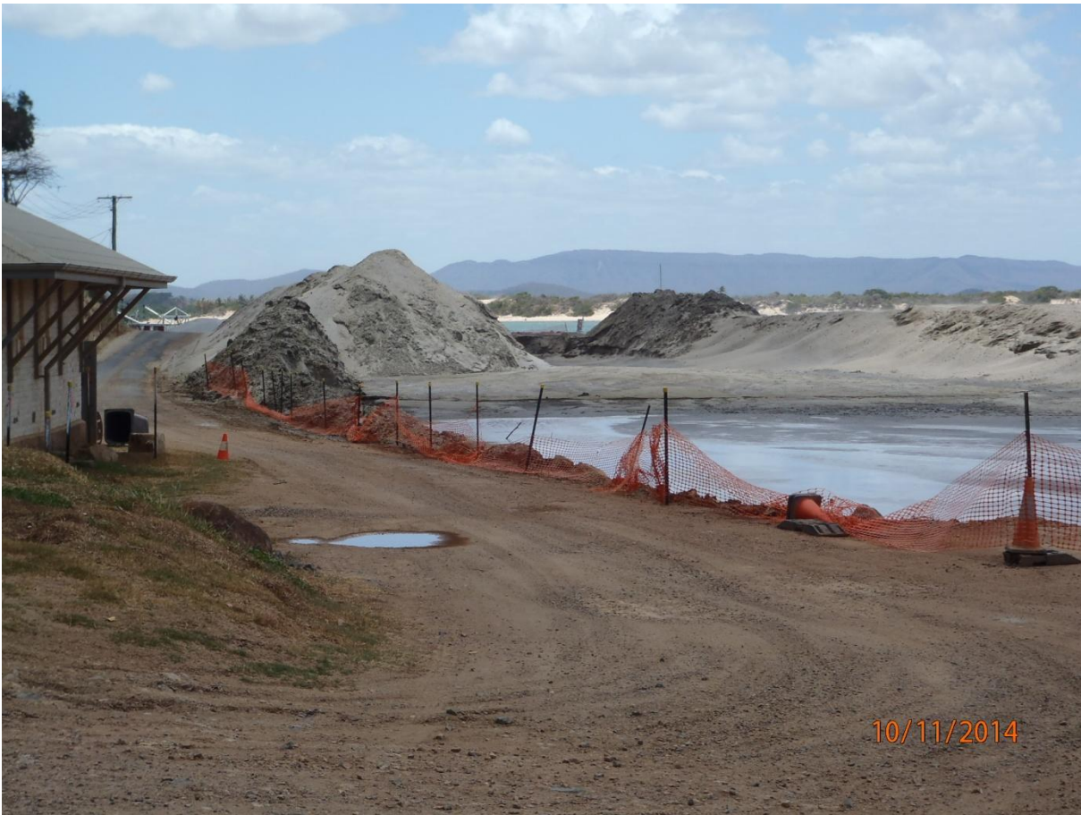
Sand pumping progress 10/11/2014
