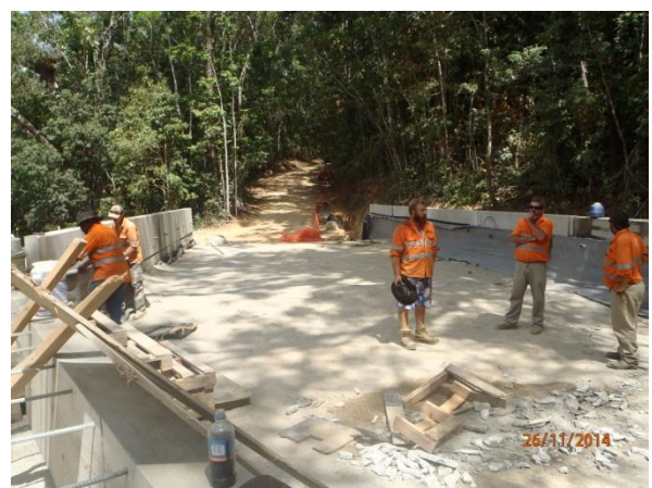
Cairns side approach, stabilised sand in place
