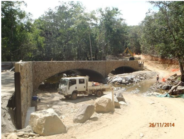
Cairns side approach-2 more sets of panels req'd to complete Cairns side windwalls
