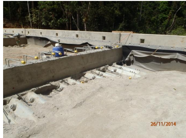
Sheerwalls and stabilised sand in place, approx 900mm more stabilised sand required Scuppers and grommets to connect reinforcing to deck slab not included in original plans
