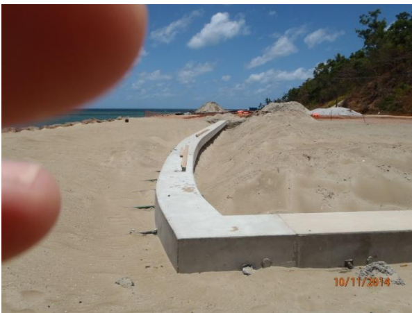
Tidal pool concrete capping completed
