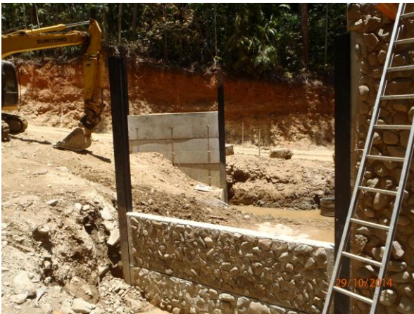
Cooktown side wingwalls
