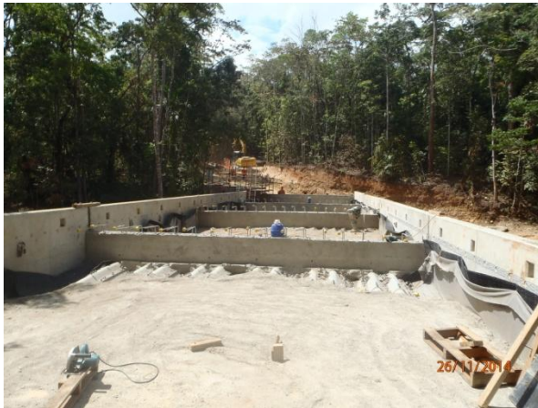
Sheerwalls and stabilised sand in place, approx 900mm more stabilised sand required Scuppers and grommets to connect reinforcing to deck slab not included in original plans
