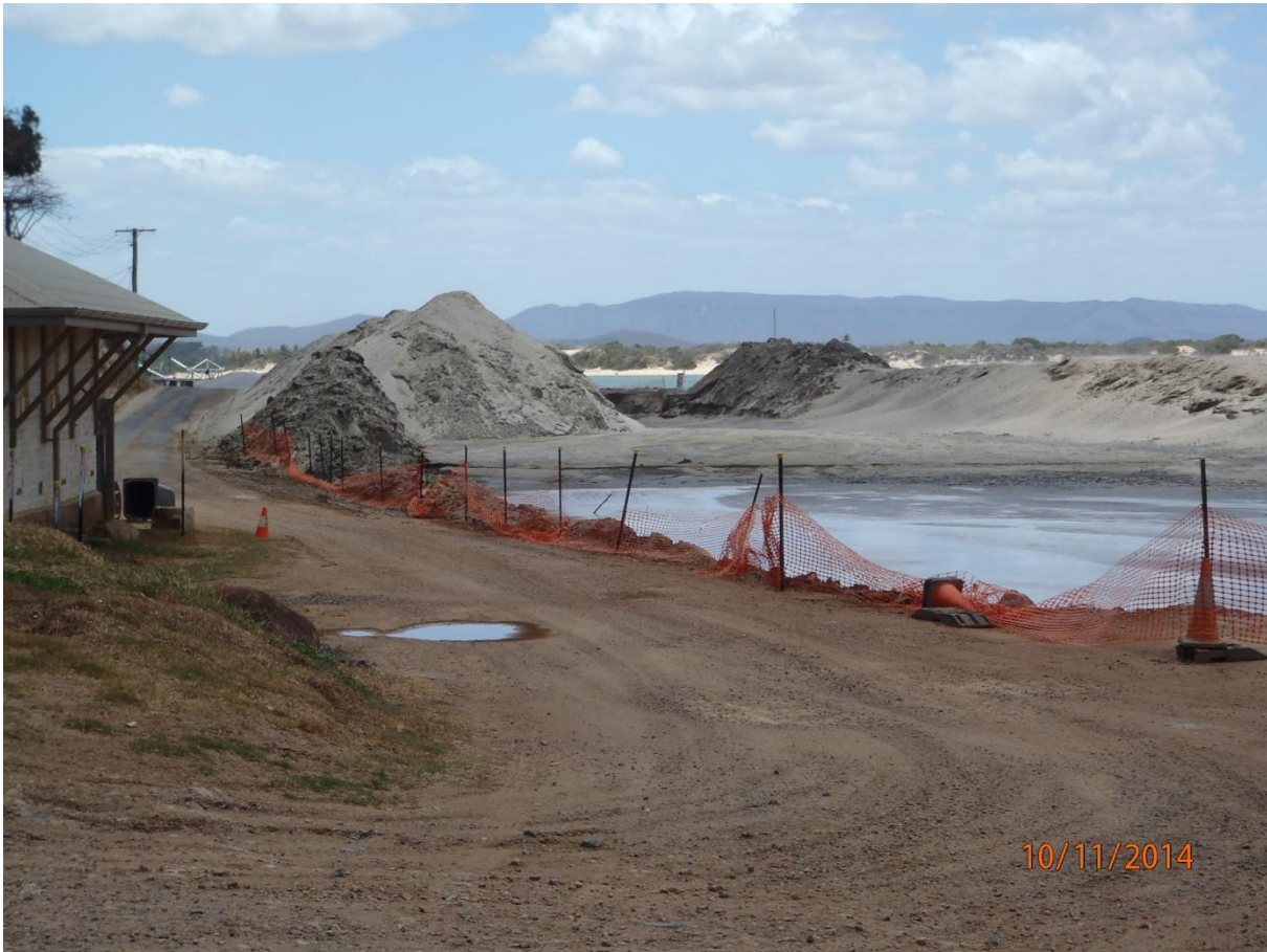
Sand pumping progress 10/11/2014
