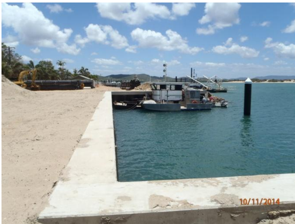
Boat Pen concrete capping completed
