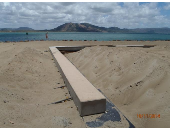
Tidal pool concrete capping completed
