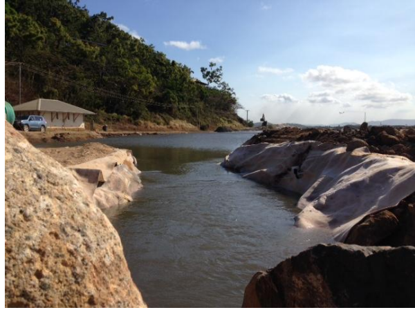
Drain through rock wall to lower water levels when backfilling
