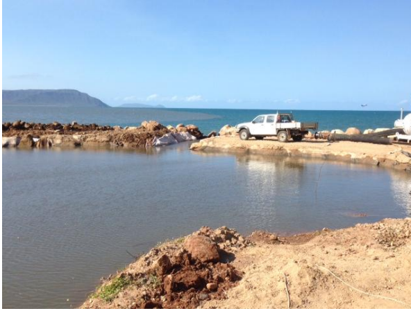
Drain through rock wall to lower water levels when backfilling
