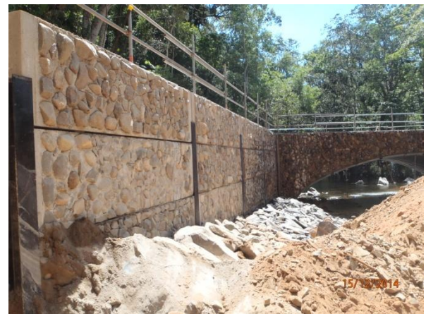
Cairns side approach showing wingwall with rock protection to footing
