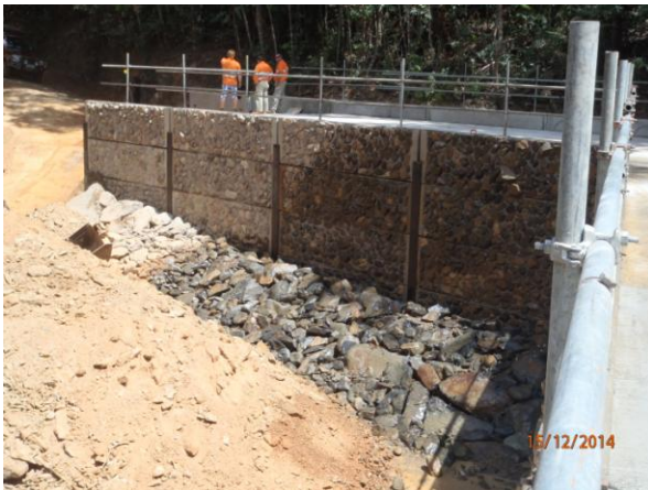
Cairns side approach showing wingwall with rock protection to footing
