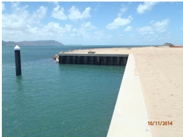
Boat Pen concrete capping completed
