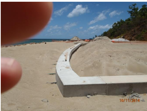
Tidal pool concrete capping completed
