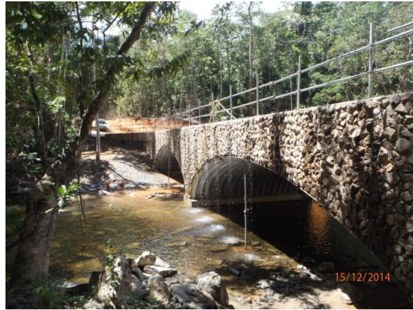
Upstream view of Cooktown approach
