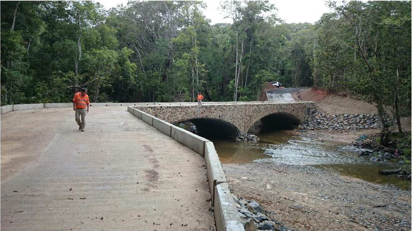
Pavement Deck Complete
