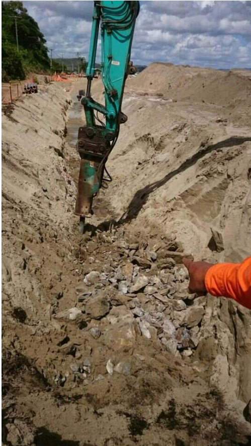
Excavation hole at end of sheet pile
