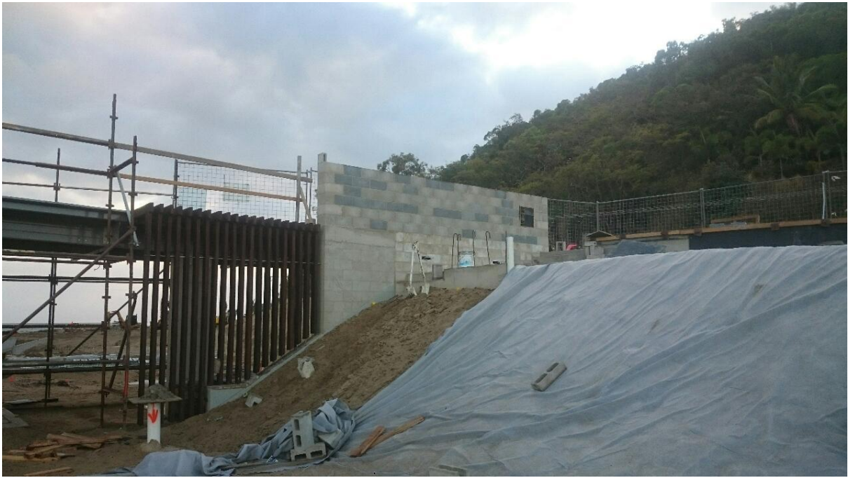
View Mound Stairs Top & Bottom
