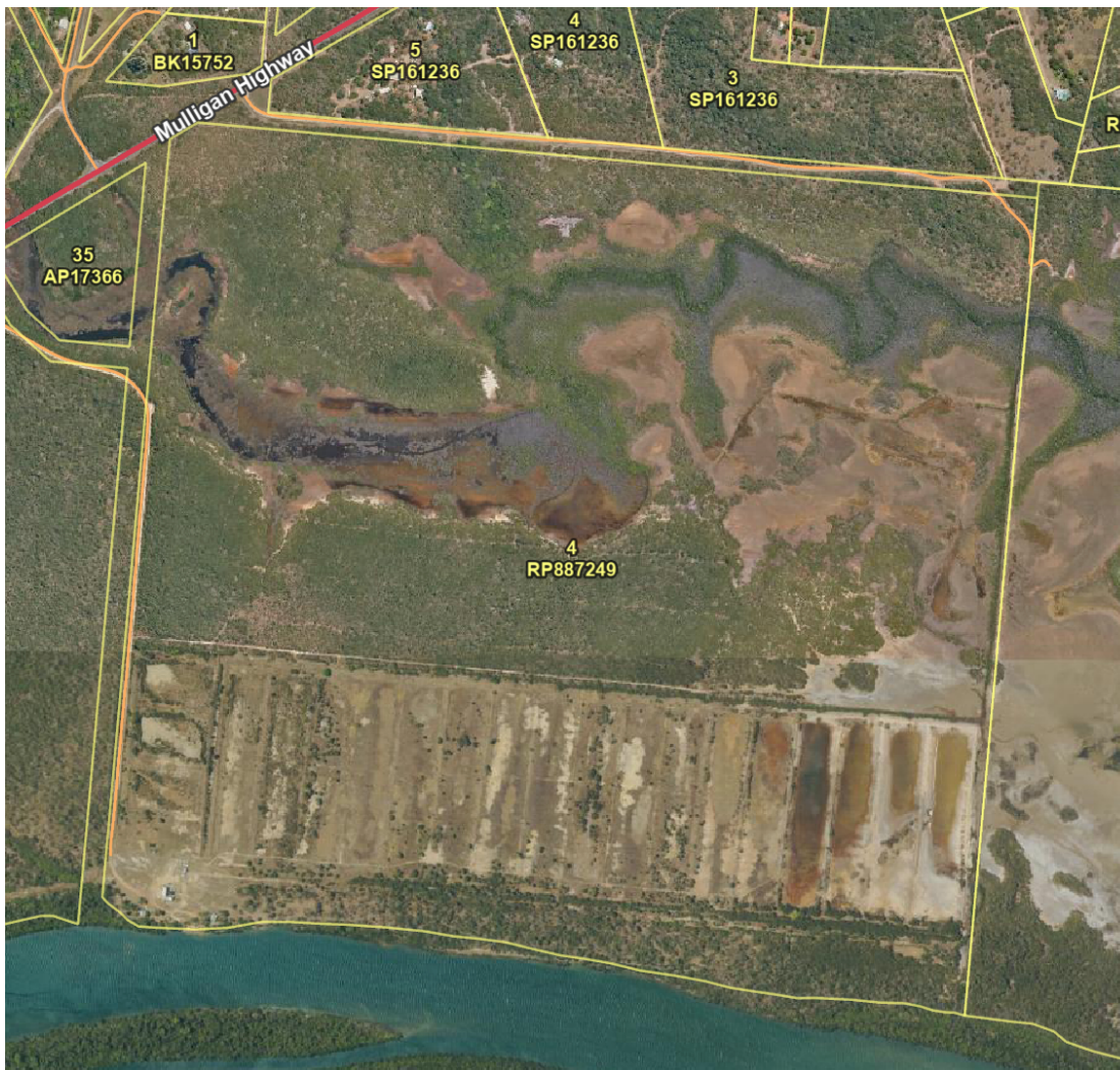
Figure 1: Aerial View of the Subject Land Parcel
