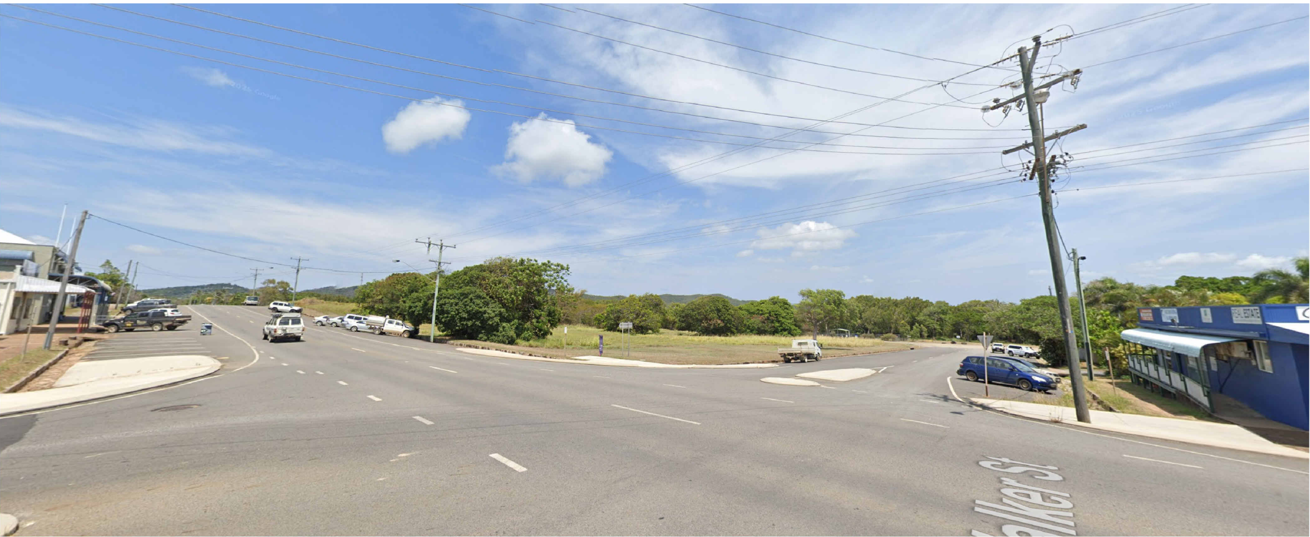
2 - Junction of Charlotte Street and Walker Street
