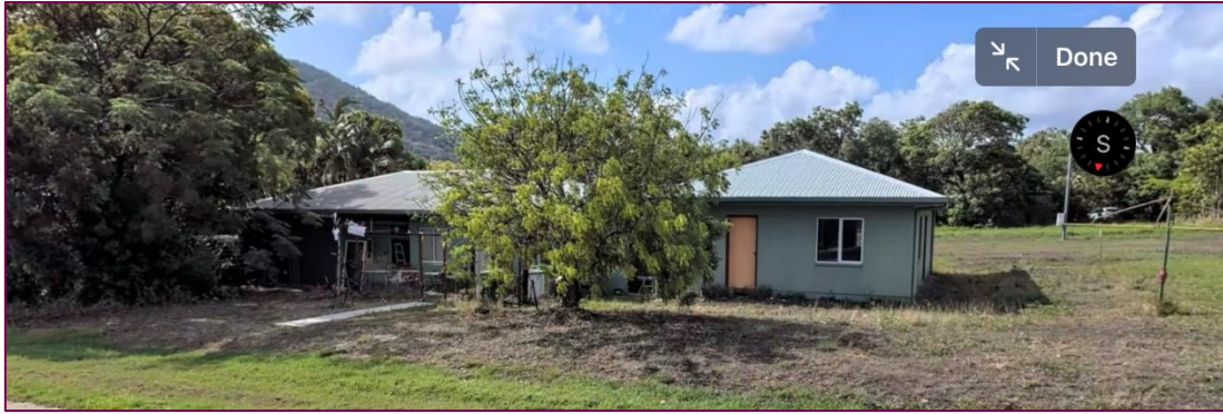
Figure 2 Howard Street Frontage
