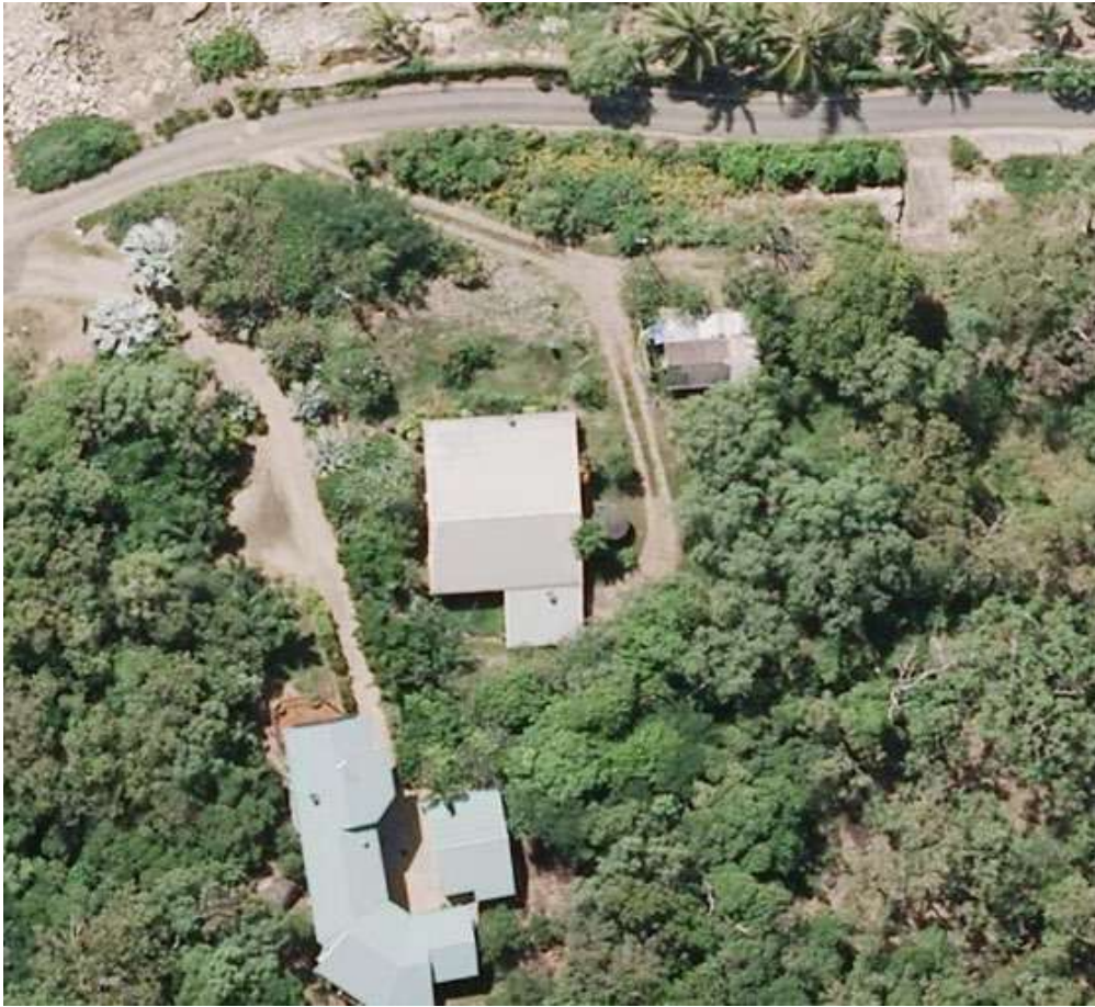
FIGURE 1 – View of Site (May 2011)
